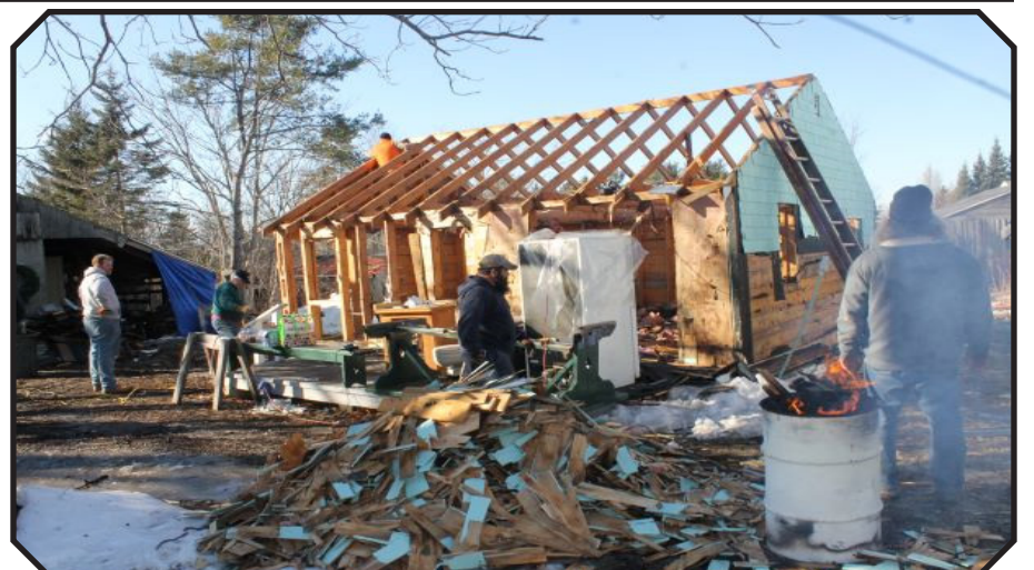
Tim's house being brought down by the Knights of Columbus of Barrington, Rhode Island. Photo credit: Eugene Hirst, Volunteer Master Photographer
