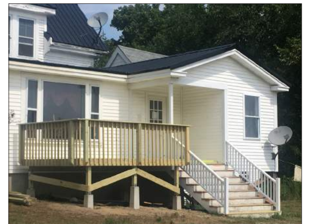
A new deck at The Sister Barbara Hance House
