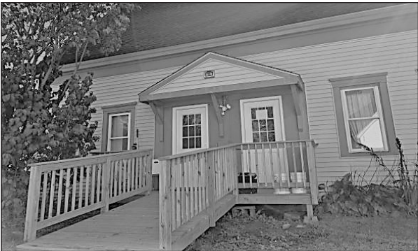
A new porch with a wider ramp was constructed for the front entrance.
