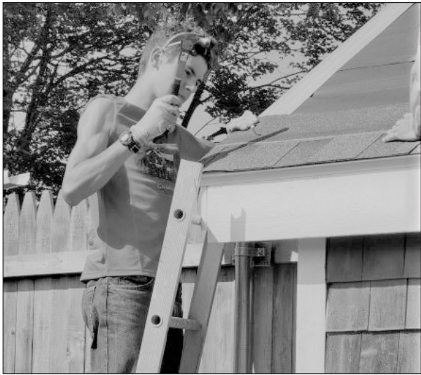
Volunteer, Owen Correll, finishes off the first row of shingles on the Special Programs Shed.
